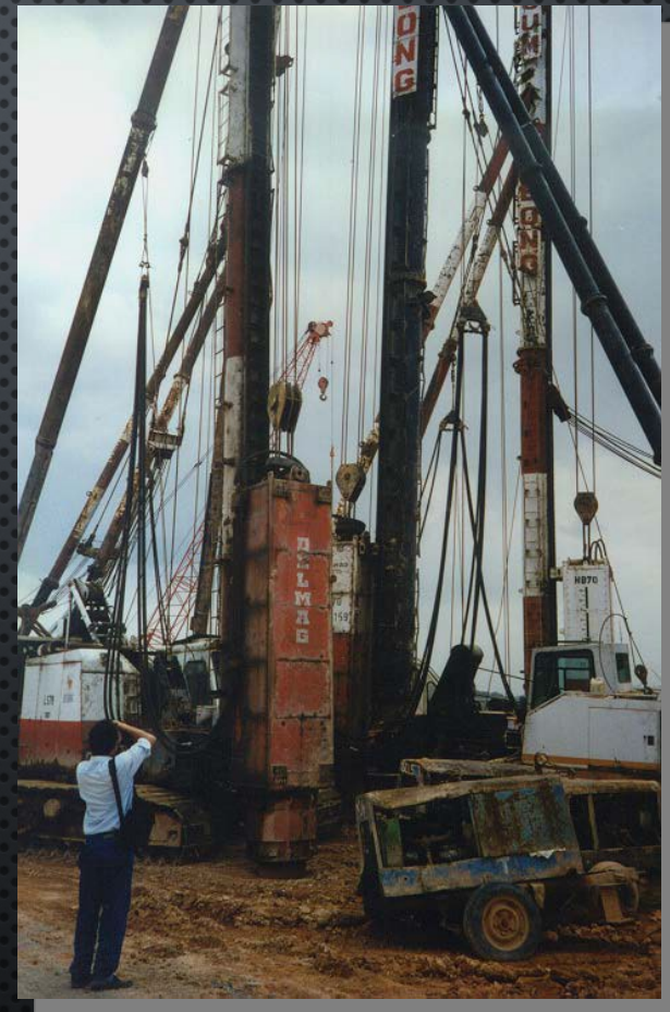
Delmag with sound proofing
