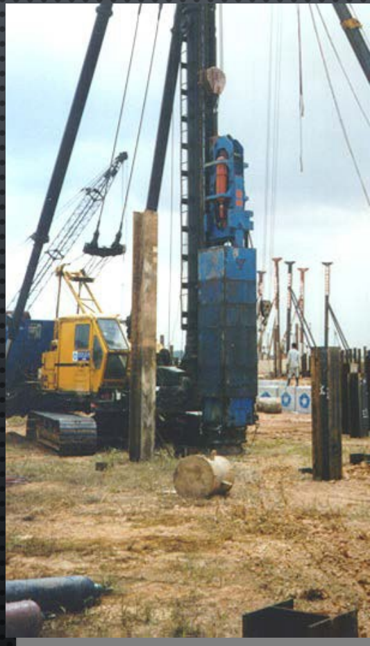
BSP with sound proofing
