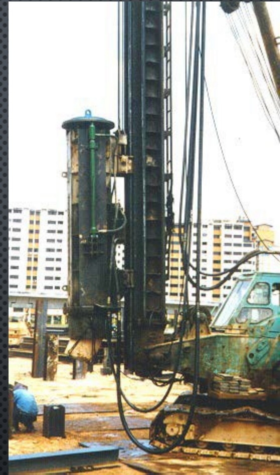
Hydroquip lowhead room manufactured in Singapore
